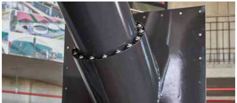
Pipe-in-pipe connection with modular link seal: Allows installation without welding and easy, maintenance-friendly replacement of the feed pipe in the digester.
