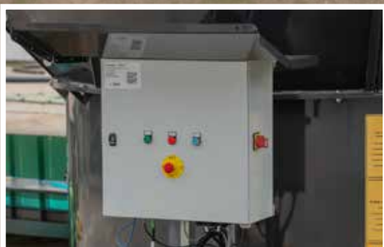
Control cabinet with rain protection
