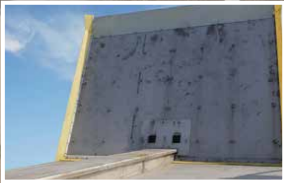
Sliding floor and push-off wall made of V2A stainless steel with PU sealing strips
