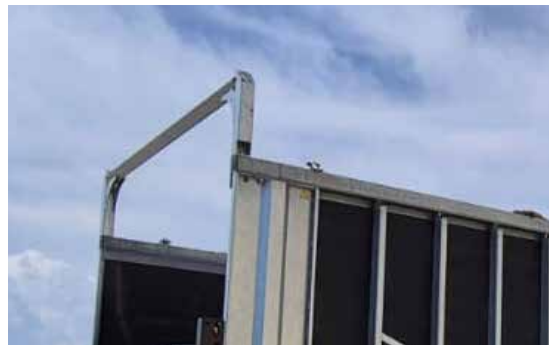
Braces to stabilize the walls
