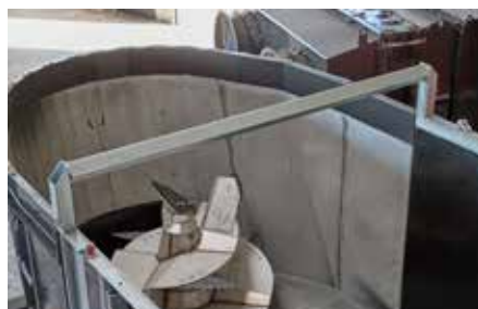
Struts to stabilise the walls
